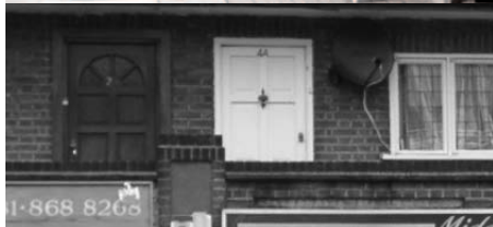
Inappropriate small scale alterations to residential flats
