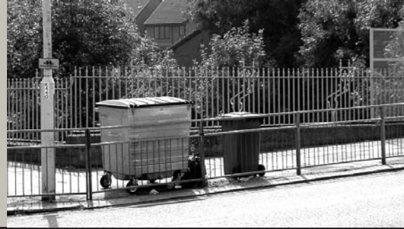
Good railings by tube line
